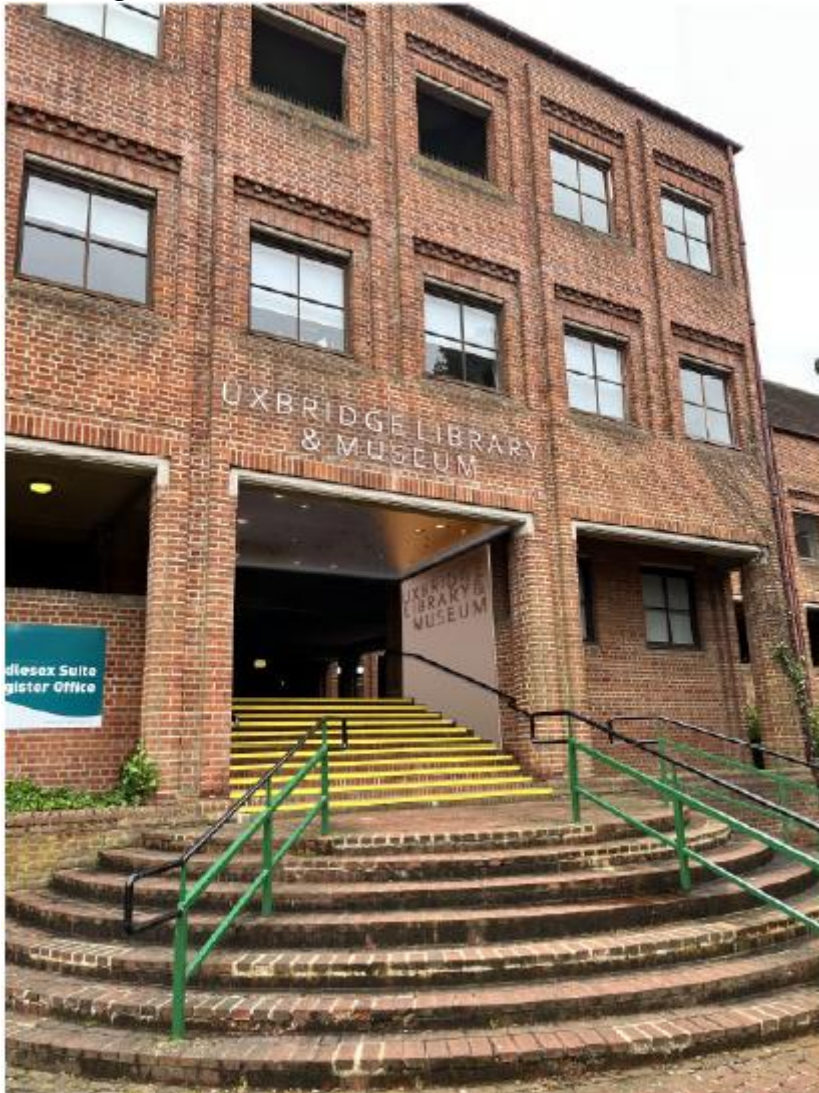
Figure 4: Proposed Signage at the Front Elevation of the Grade II Listed Building.
