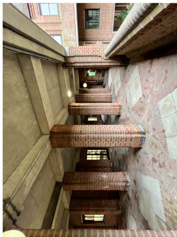
Collonade existing view
